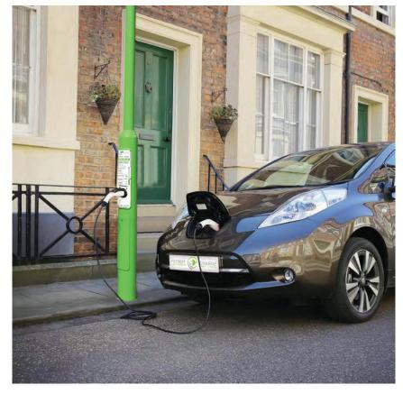
There are hundreds of thousands of street lights throughout the UK, many of which have sufficient electricity available to be upgraded to provide electric vehicle charging.
